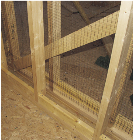
Example of insulation netting support and timber cross bracing
