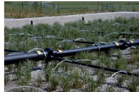
Figure 5-6: Vertical sand filter
