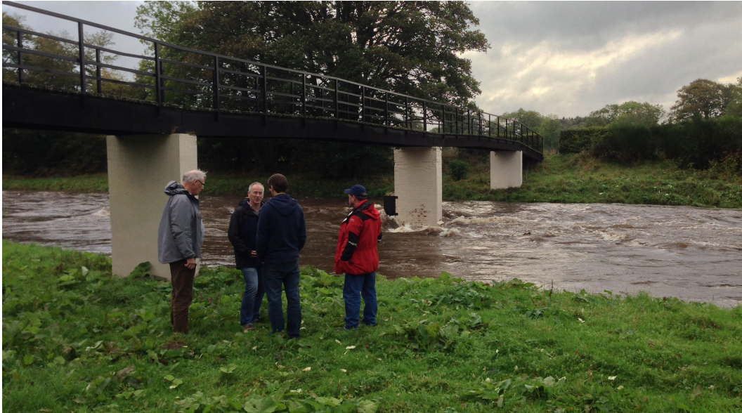
Figure 5.16. South Esk footbridge, a potential counter site for River South Esk. A footbridge downstream of the South Esk weir site. Photo courtesy of InStream Fisheries Research.
