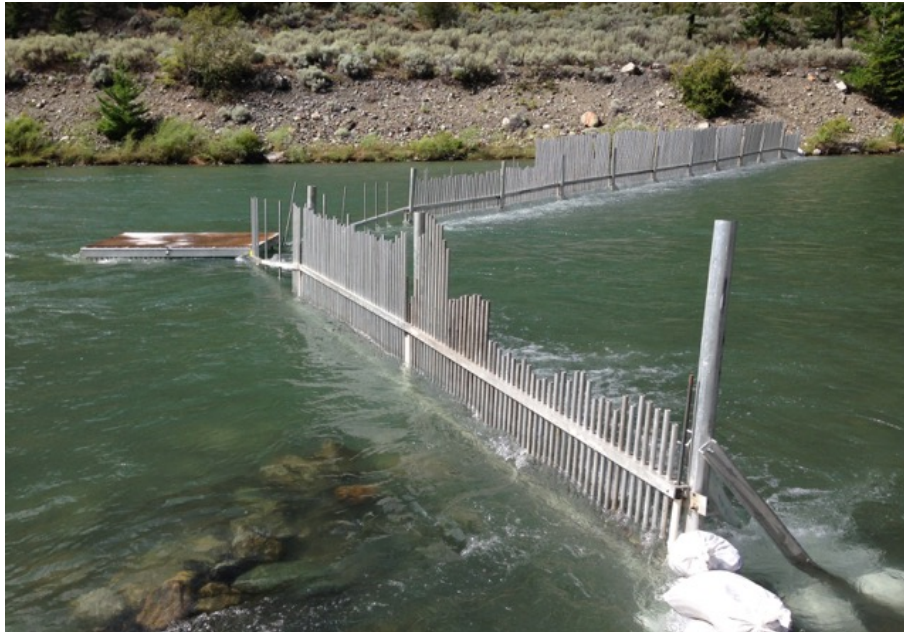
Figure 2.11. Seton River picket fence with trap box. River width approximately 30 m, discharge 30 m 3 /s, depth 1 m. Photo courtesy of InStream Fisheries Research.
