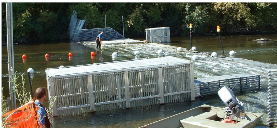
Figure 2.9. Alaskan floating fence used on the Stanislaus River, United States. Panels are 20 ft. long and incorporate a Vaki counter unit. Photo courtesy of Vaki.
