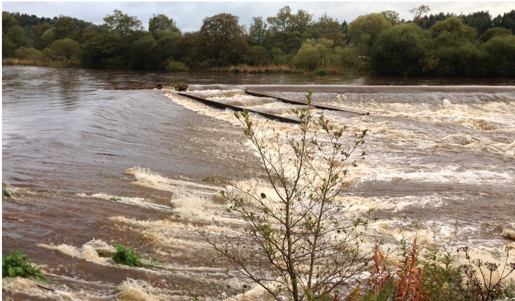
Figure 5.15. South Esk weir, a potential counter site for River South Esk. A small fish pass exists in the middle of the fish weir. Photo courtesy of InStream Fisheries Research.
