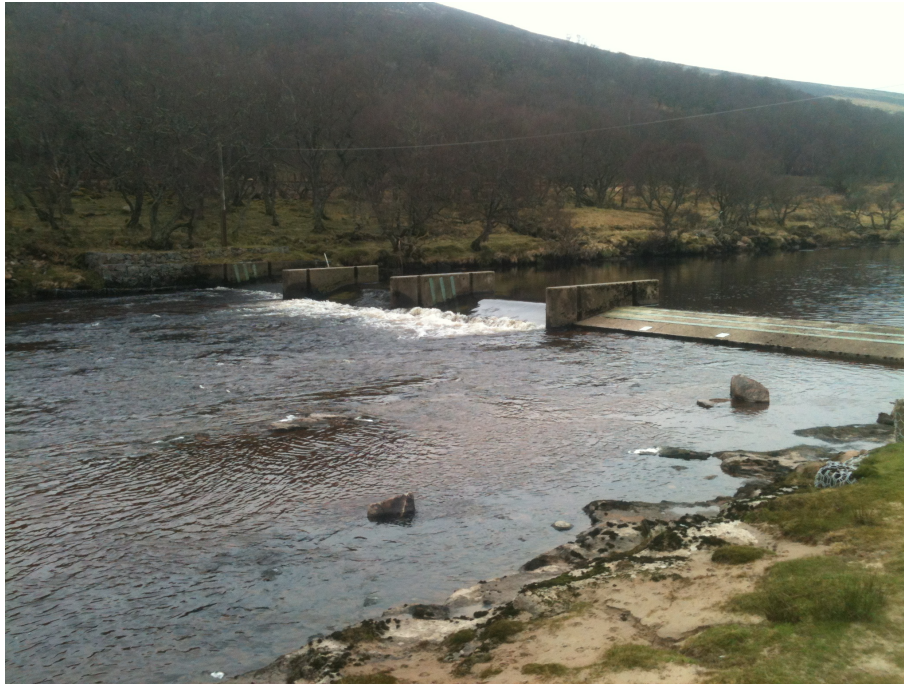
Figure 2.14. Helmsdale resistivity fish counter weir with four channels at low flow. Photo courtesy of InStream Fisheries Research.
