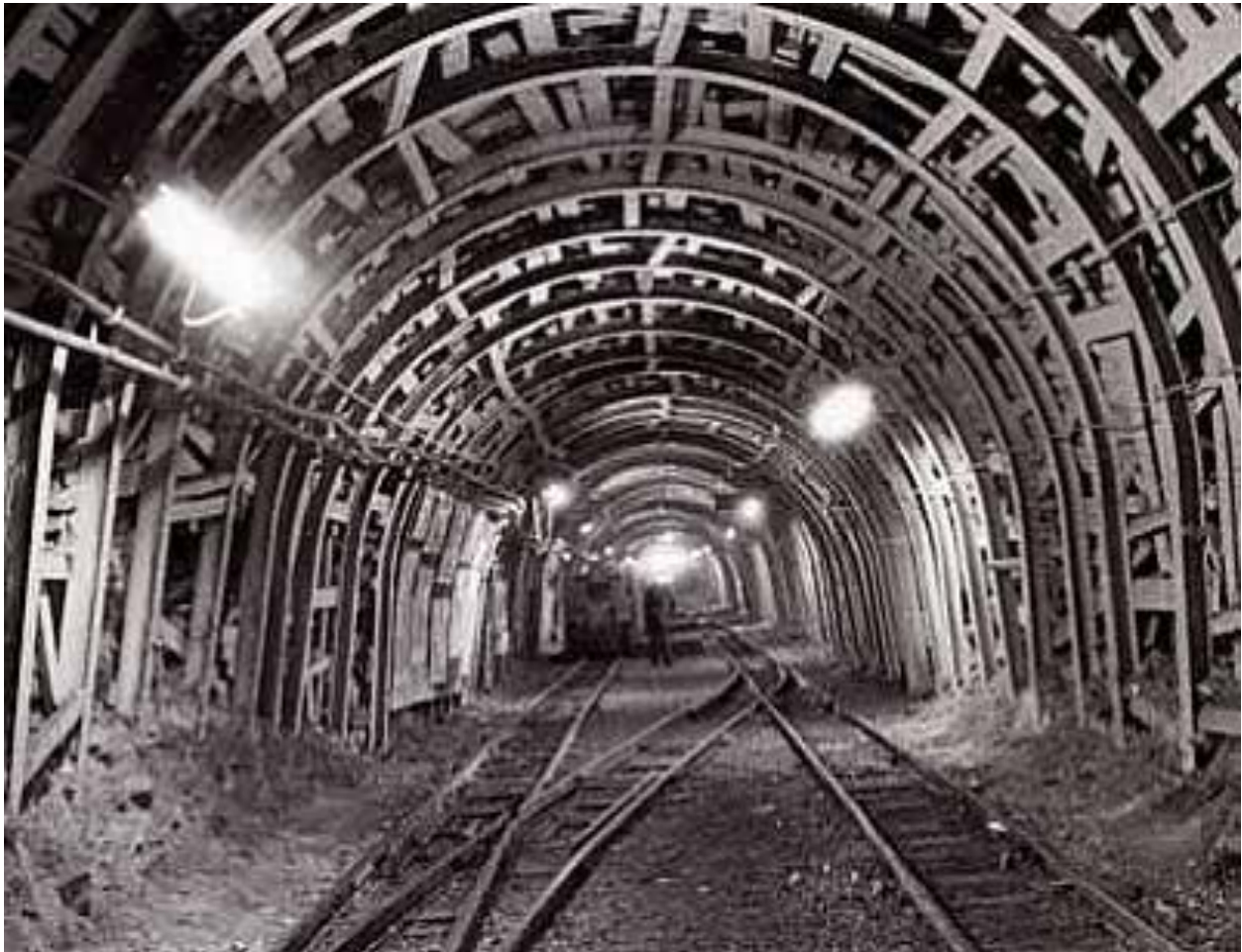
Figure 23 Monktonhall Colliery Underground Roadway: view looking along an underground roadway at Monktonhall Colliery, Midlothian, 1970s. This colliery produced coal from 1967 to 1997. Image courtesy of the Scottish Mining Museum.
