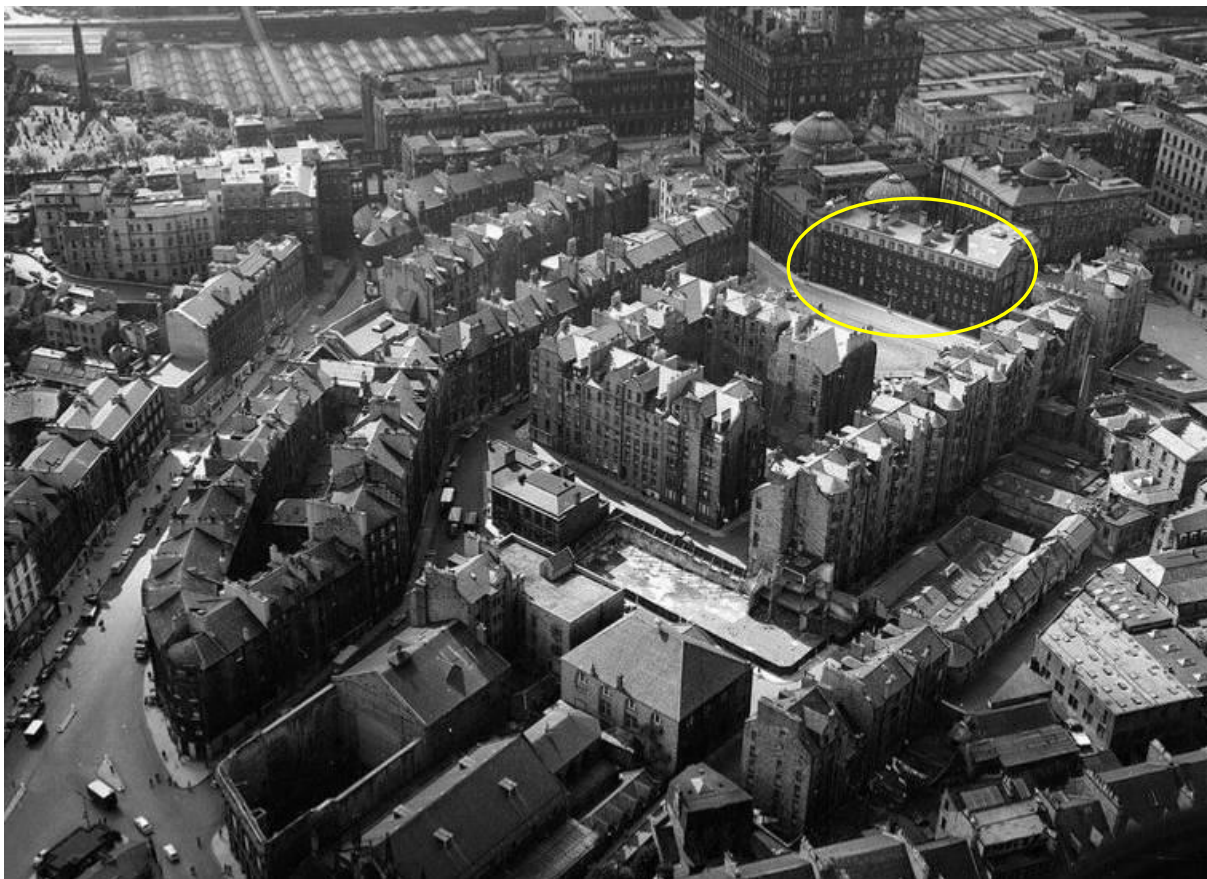
1958 aerial photograph of St James Square prior to partial demolition in 1970 for St James Centre development
