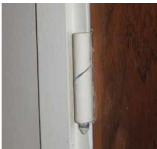
Figure 5 Rising butt hinge
