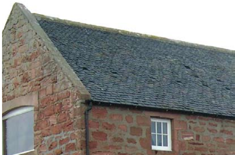
Illus 3.14.6 Flush roof vents (Photo: D Urquhart).
