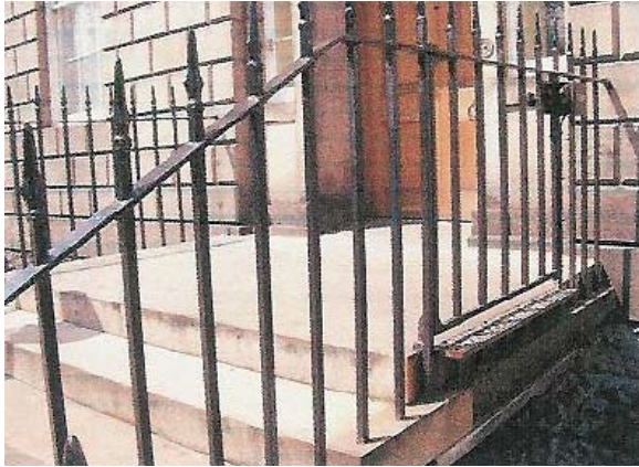
Illus 4.1.4 Access to platform lift installed at Bute House, Edinburgh. Note the reuse of iron railings to form the access gate to the lift. (Photo: NTS).
