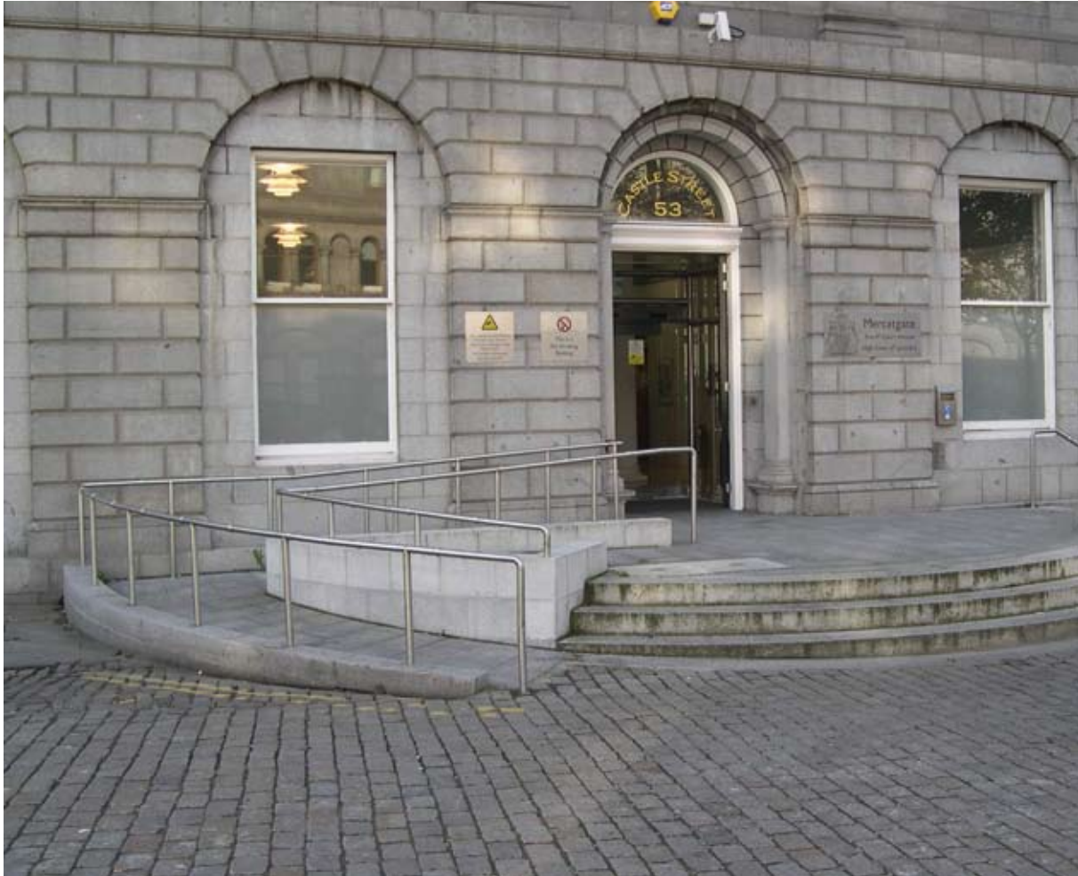
Illus 4.1.3 Sympathetically designed access ramp and steps to 1801 Category A listed converted bank building (Photo: D Urquhart).
