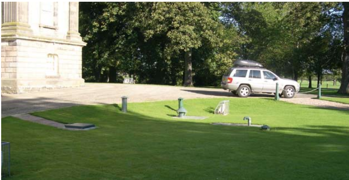
Illus 2.13.1 Landscaped underground storage tank with minimal intrusion into historic landscape which could have been improved with more careful detailing of intrusions. (Photo: D Urquhart).
