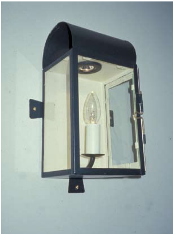
Illus 2.10.1 Emergency lighting installation in a listed Category A building (Photo: S Brown).
