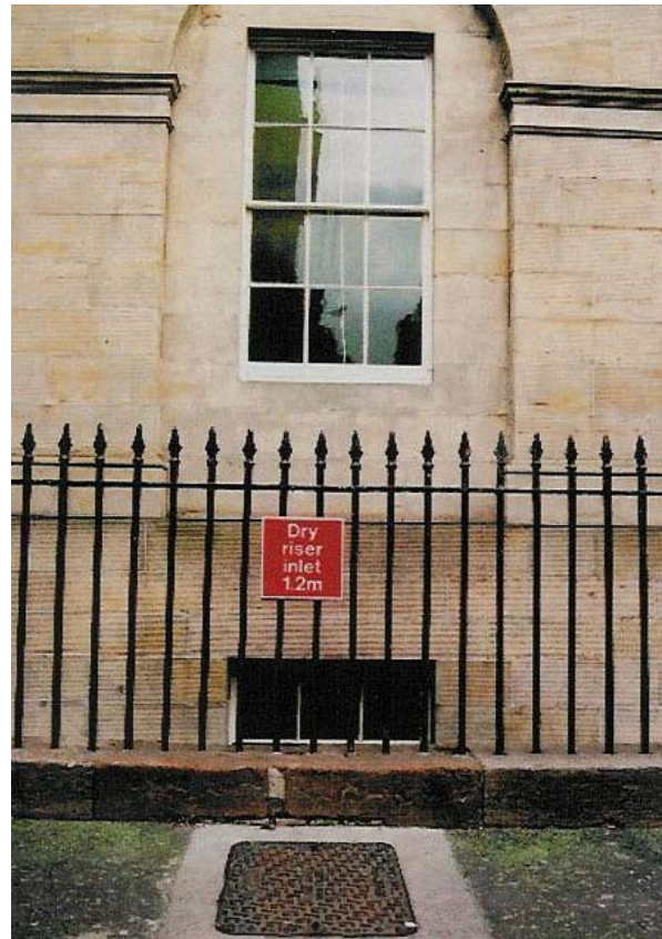
Illus 2.14.1 Dry riser inlet located to reduce impact on historic character by locating inlet valves beneath cast iron cover in footpath (Photograph from TAN 28: Paul Beaton, Historic Scotland).
