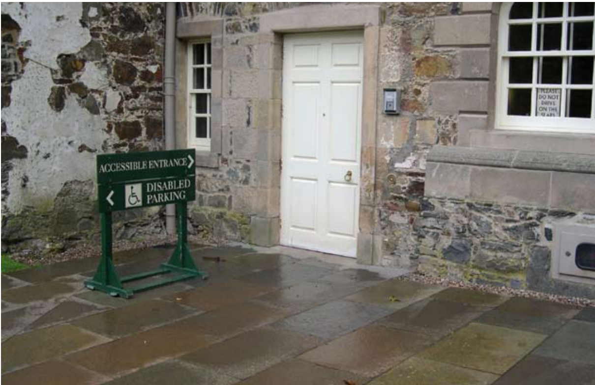
Illus 4.1.1 Natural stone paving forming access for disabled people to Duff House (Photo: D Urquhart).
