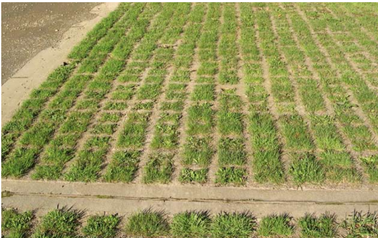
Illus 2.12.1 Improvement to fire service access at Duff House. A hard standing and turning area for fire service vehicles has been formed using ‘Grass-crete’ to reduce impact on the historic landscape. (Photo: D Urquhart).
