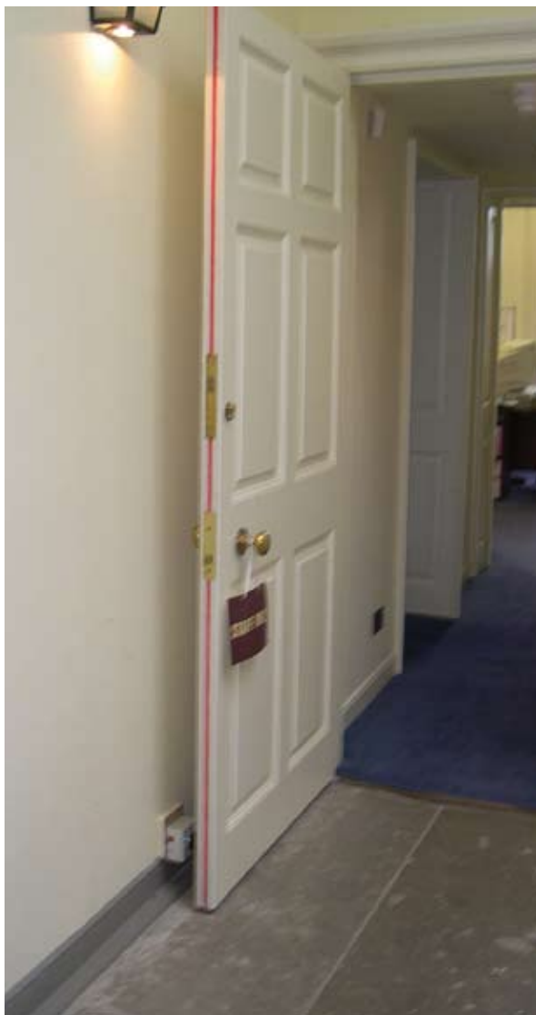
Illus 2.9.1 Hold open device on historic paneled door within an escape route (Photo: D Urquhart)
