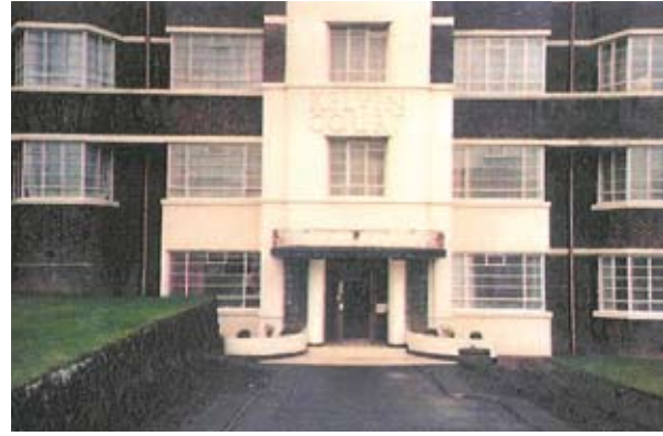
Illus 3.14 Early C20 listed Category B apartment building with steel windows. (Photo: Historic Scotland).
