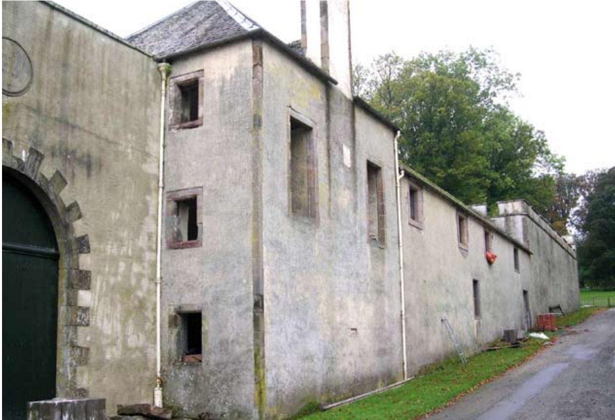
Illus 3.2 Sympathetic conversion of former storage building at Foulis Castle into a family home with rubble walls lime harled, with sandstone facings to openings (Photo: D Urquhart).
