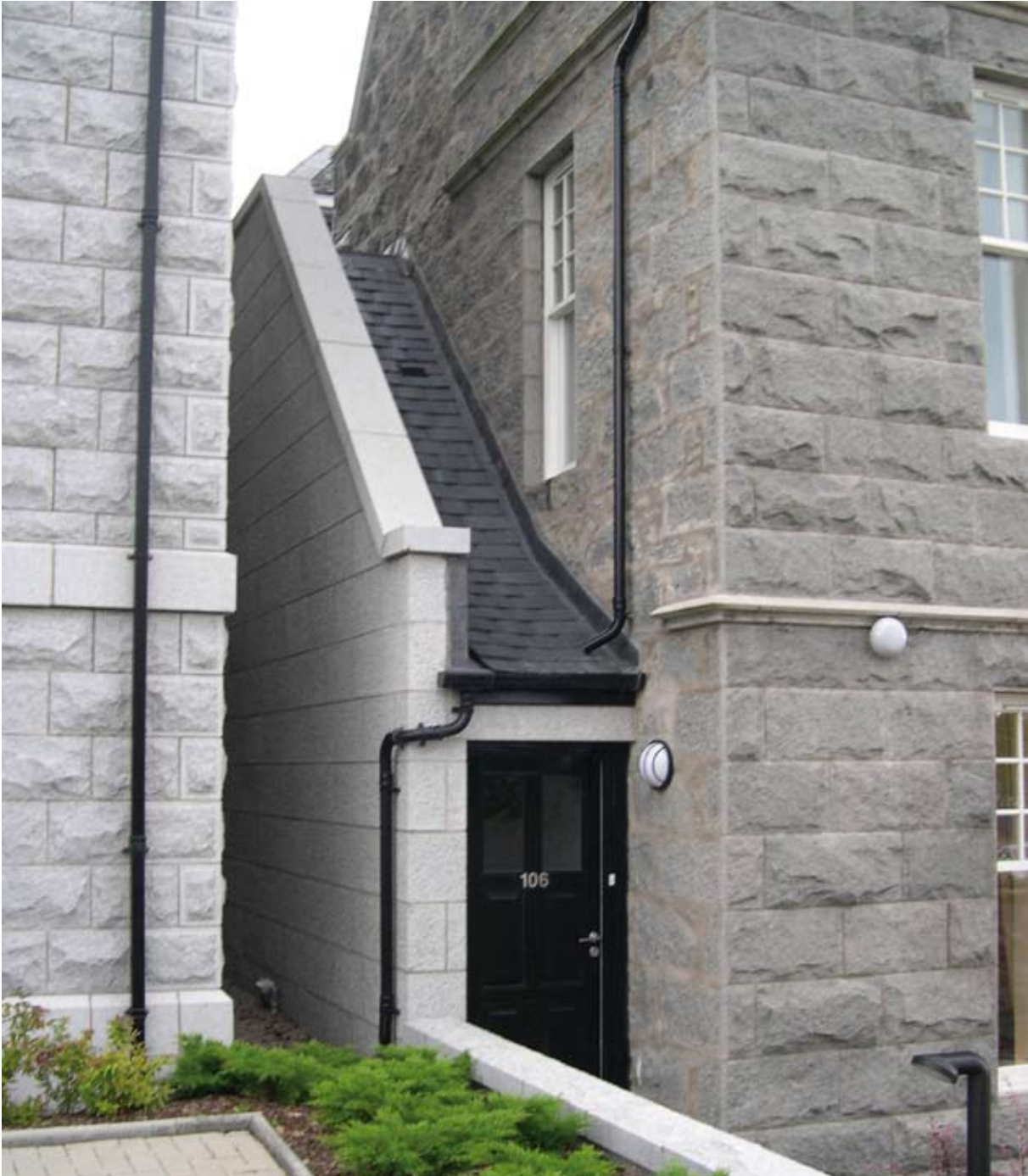
Illus 3.17 New entrance to an upper floor apartment listed Category B former hotel. The new wall is in imported granite (as is the new building to the left) rather than the rock-faced Kemnay granite of the original wall. (Photo: D Urquhart).
