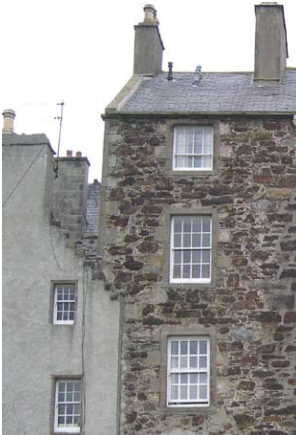
Illus 3.15(a), (b) Replacement PVCu double glazed sash and case window (bottom window in exposed rubble wall). While resembling the timber sash and case window above, the wider frame and glazing bars detract from the character of this Category B listed building (1790) converted into apartments. (Photo: D Urquhart).
