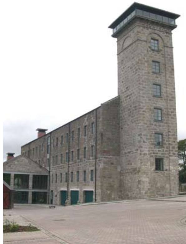
Illus 2.4 Former spinning mill (listed Category A) converted into apartments. An important issue in the conversion was the unique cast-iron structural system. The extension to the side with large glazed areas is a restaurant cut back from a bigger shed. The glass belvedere replaced a long-missing cupola for a water tank and bell (Photo: D Urquhart).
