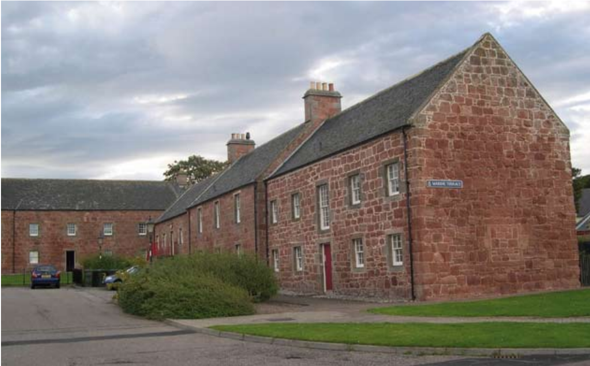
Illus 3.9 Traditional Scottish sandstone rubble wall. Conversion of former hemp works (Photo: D Urquhart).
