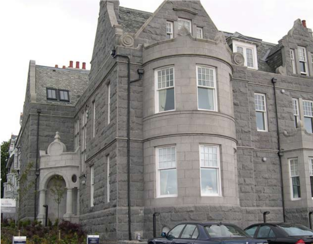
Illus 3.18 View of the main entrance elevation of the conversion shown in Illus 3.17. (Photo: D Urquhart).
