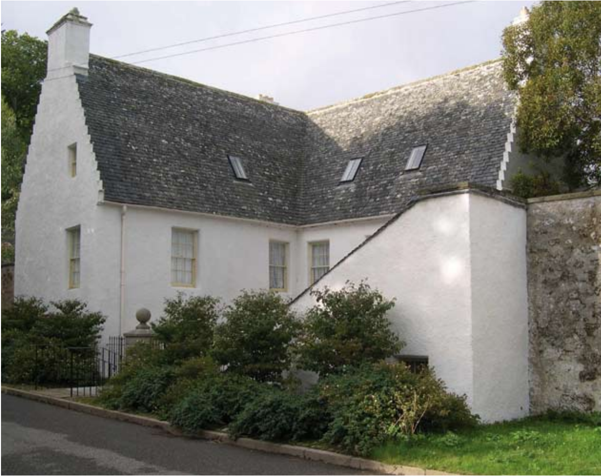
Illus 3.12(b) Good example of recent lime coating on a restored Category A listed building. (Photo: D Urquhart). Note the new DPC below the garden wall cope.
