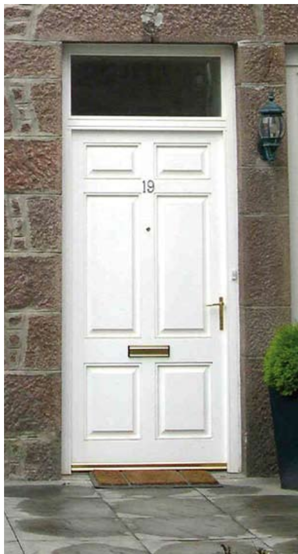
Illus 3.16(a) The door on the left is an inappropriate modern replacement plastic door in this traditional 1914 building (Photo: D Urquhart).
