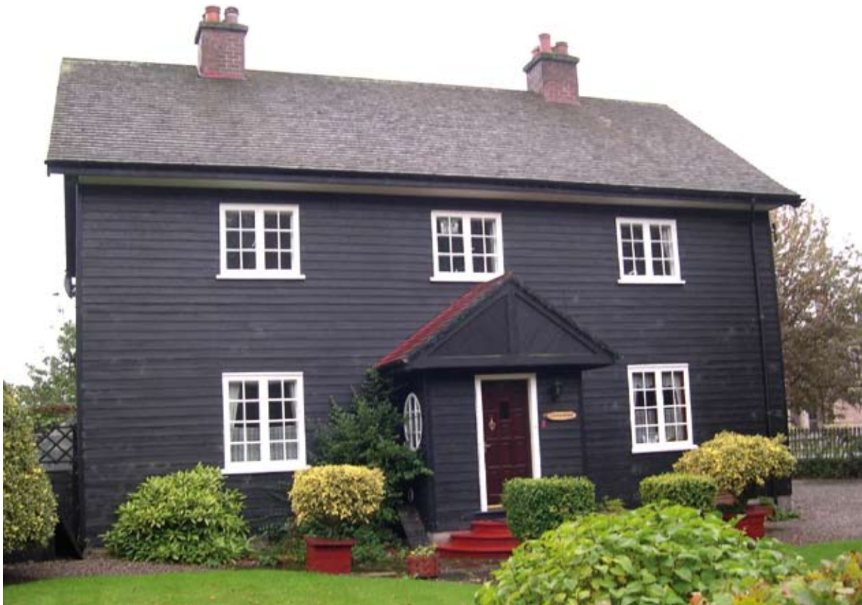
Illus 3.7 Well-maintained, single-skin timber framed house (Photo: D Urquhart).
