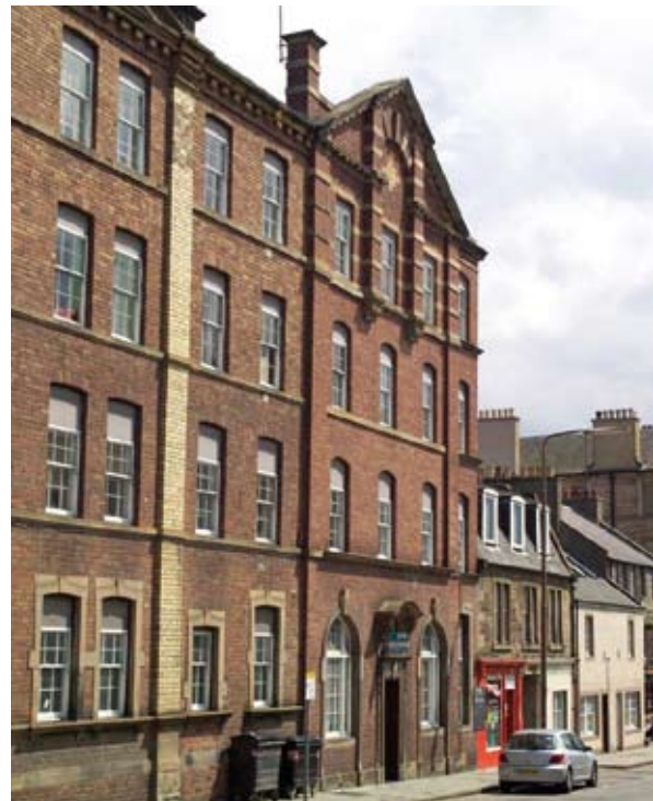
Illus. 1.2. An example of an unlisted former printing works that has been converted into apartments. Identically-sized windows have been installed in openings of variable dimensions below false ceilings fronted by an off-white infill. Fully-glazed openings might have been preferred, with false ceilings set back from these, or even given a dark reflective finish, had the building been listed and/or advice requested from Historic Scotland (Photo: Historic Scotland).
