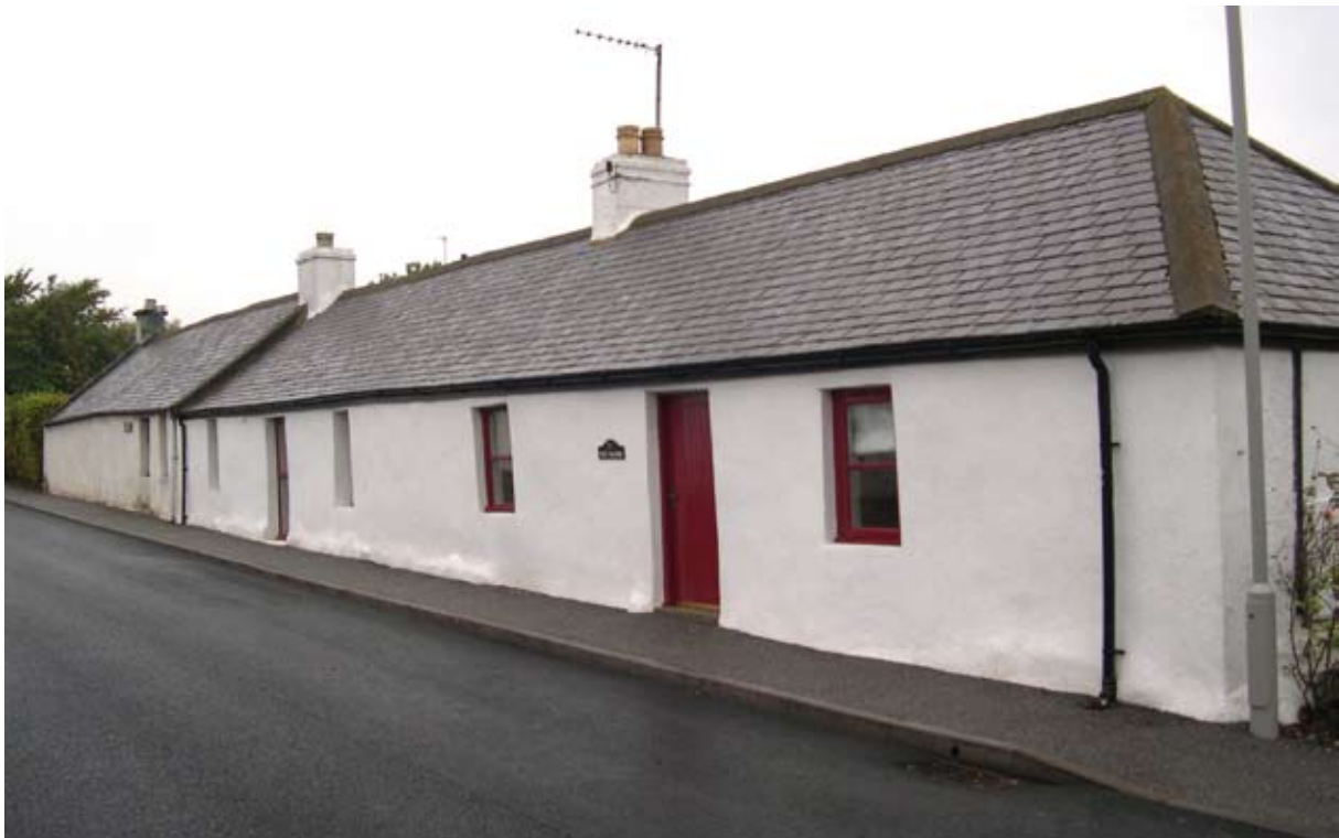
Illus 3.3 Clay and bool cottages (C(S) Listed), Morayshire. Unfortunately, now rendered with a hard cement mortar Note: boulder base course and modern slated roof, which replaces the original traditional 'clay thatch'. (Photo: D Urquhart).
