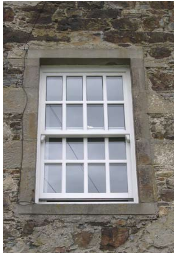
Illus 3.15(a), (b) Replacement PVCu double glazed sash and case window (bottom window in exposed rubble wall). While resembling the timber sash and case window above, the wider frame and glazing bars detract from the character of this Category B listed building (1790) converted into apartments. (Photo: D Urquhart).
