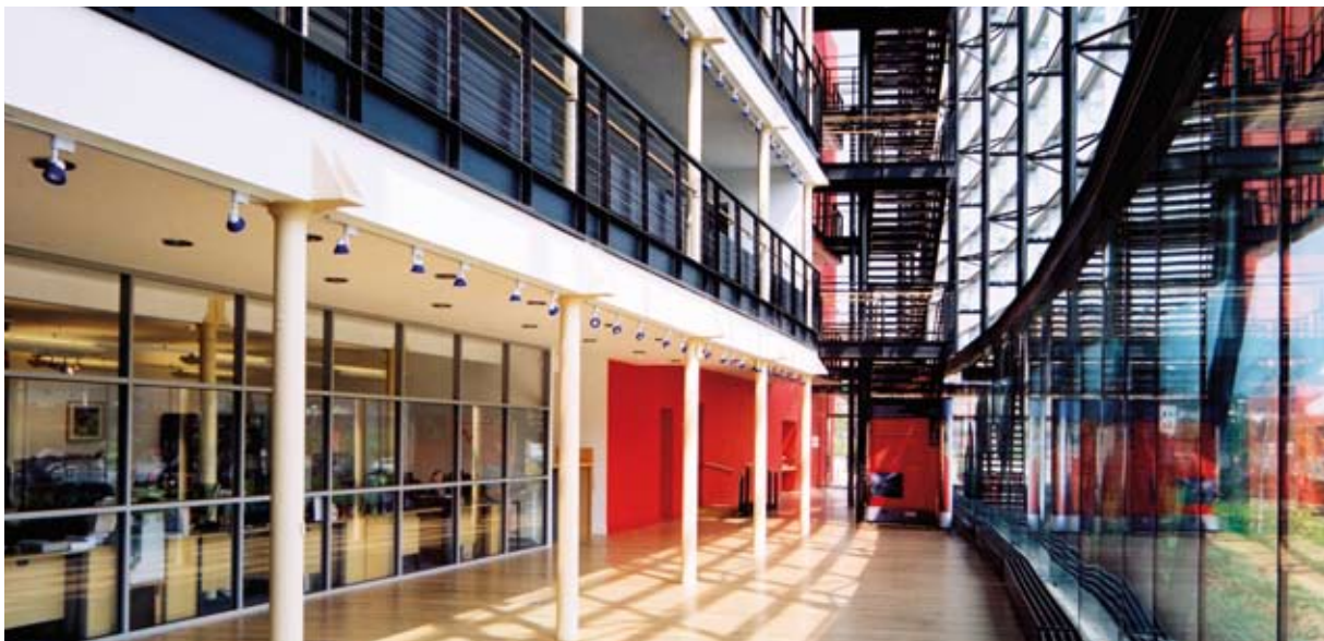
Illus 2.6a Innovative conversion of a sandstone and iron-framed building now part of a business and retail park (interior view). While the conversion of the building results in a modern, practical and economically viable development, the important historic features have been retained, as can be seen from the sandstone façade and the internal structural arrangement of columns, beams and floors. Historic columns and beams are retained behind a new façade cut across a very deep-plan yarn store. (Photographs ©Historic Scotland Photo Library).
