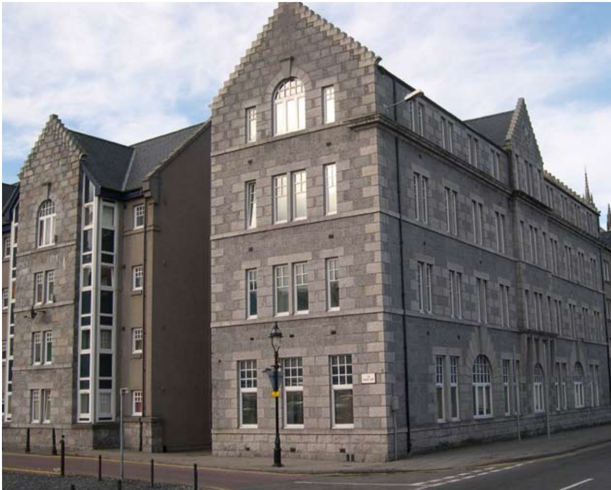
Illus 1.3 Former lodging house converted to apartments with new extension on the left (Photo: D Urquhart).
