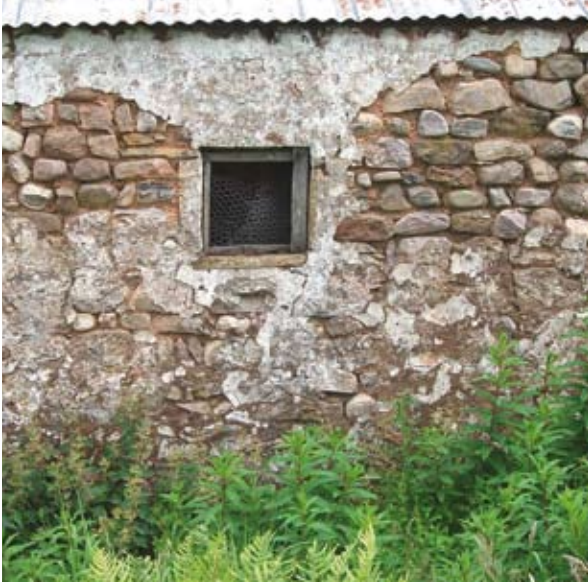
Illus 3.4 Example of a clay and boole wall, Morayshire (Photo: S Montgomery, Historic Scotland).
