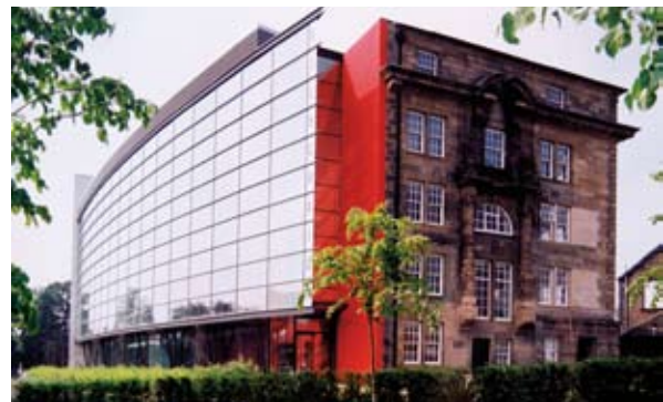
Illus 2.6b Innovative conversion of a sandstone and iron-framed building (exterior view).
