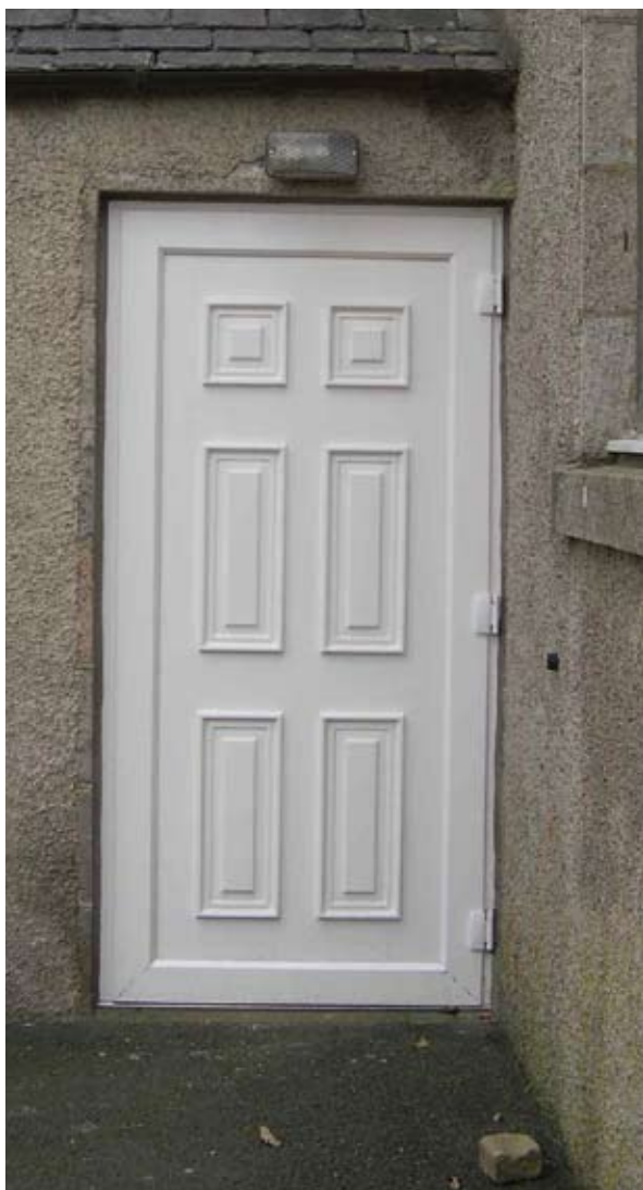
Illus 3.16(a) The door on the left is an inappropriate modern replacement plastic door in this traditional 1914 building (Photo: D Urquhart).
