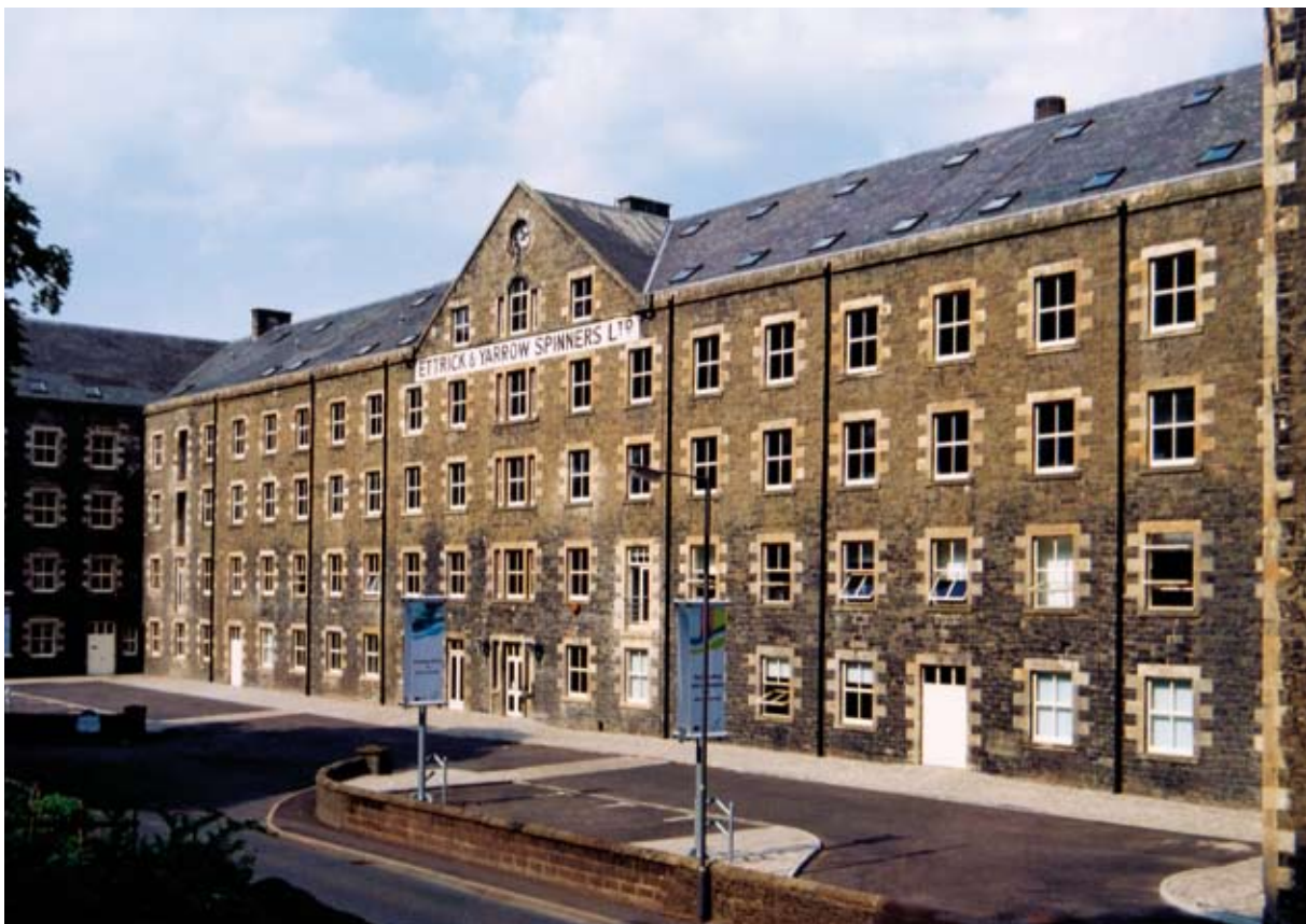
Illus 1.5 Conversion of a redundant spinning mill to a small Business Gateway by Scottish Borders Enterprise. A conservation plan guided the development (Photo: ©Crown Copyright, 2007, Historic Scotland Images).
