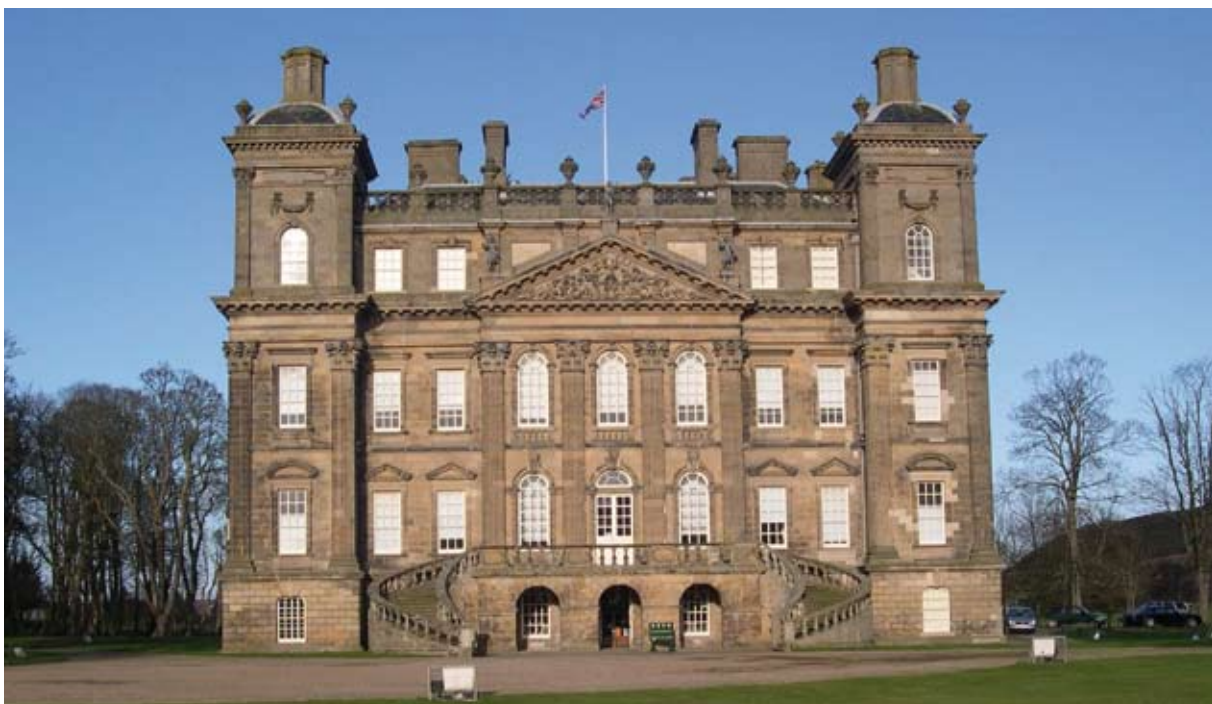
Illus 1.1 Listed Category A Duff House was rescued from a disused state and converted into a country house gallery containing art works from the National Galleries of Scotland (Photo: D Urquhart).
