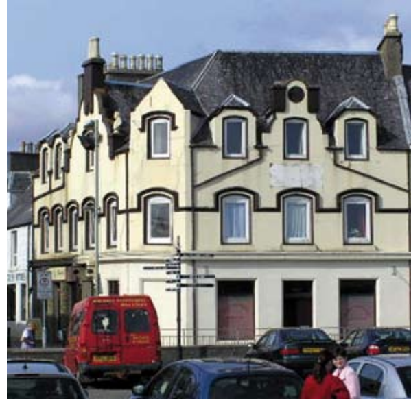
Illus 3.5 Despite its traditional appearance, this C(S) listed building (Waverley Buildings, Stornoway) is constructed from concrete. (Photo: Andrew Wright).
