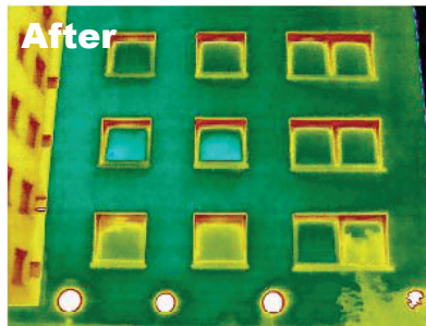
Example property – mid floor flat, cavity wall after external insulation installed. EPC-EE rating 76 (image courtesy of IRT Surveys)
