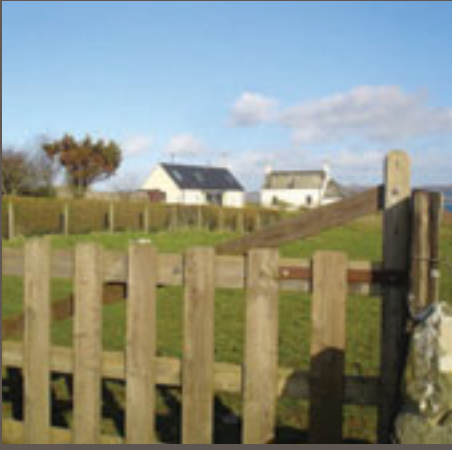
A single house fitting in next to an older house
