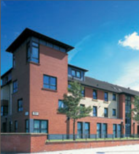
One of the later stages of Gorbals redevelopment: a simple design with a distinctive corner
