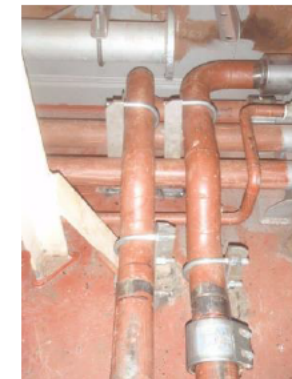
Correct Axilock Fit up Sign off CMAL/QC
