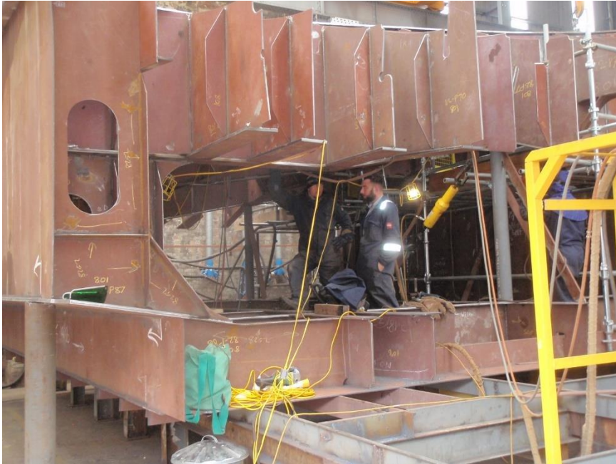
Vessel 1 – Stern Unit Under Construction
