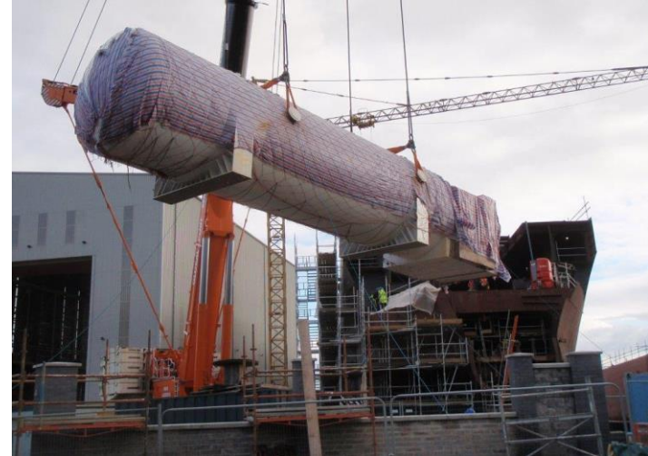
Vessel 1 – LNG Tank Lift/Shipping
