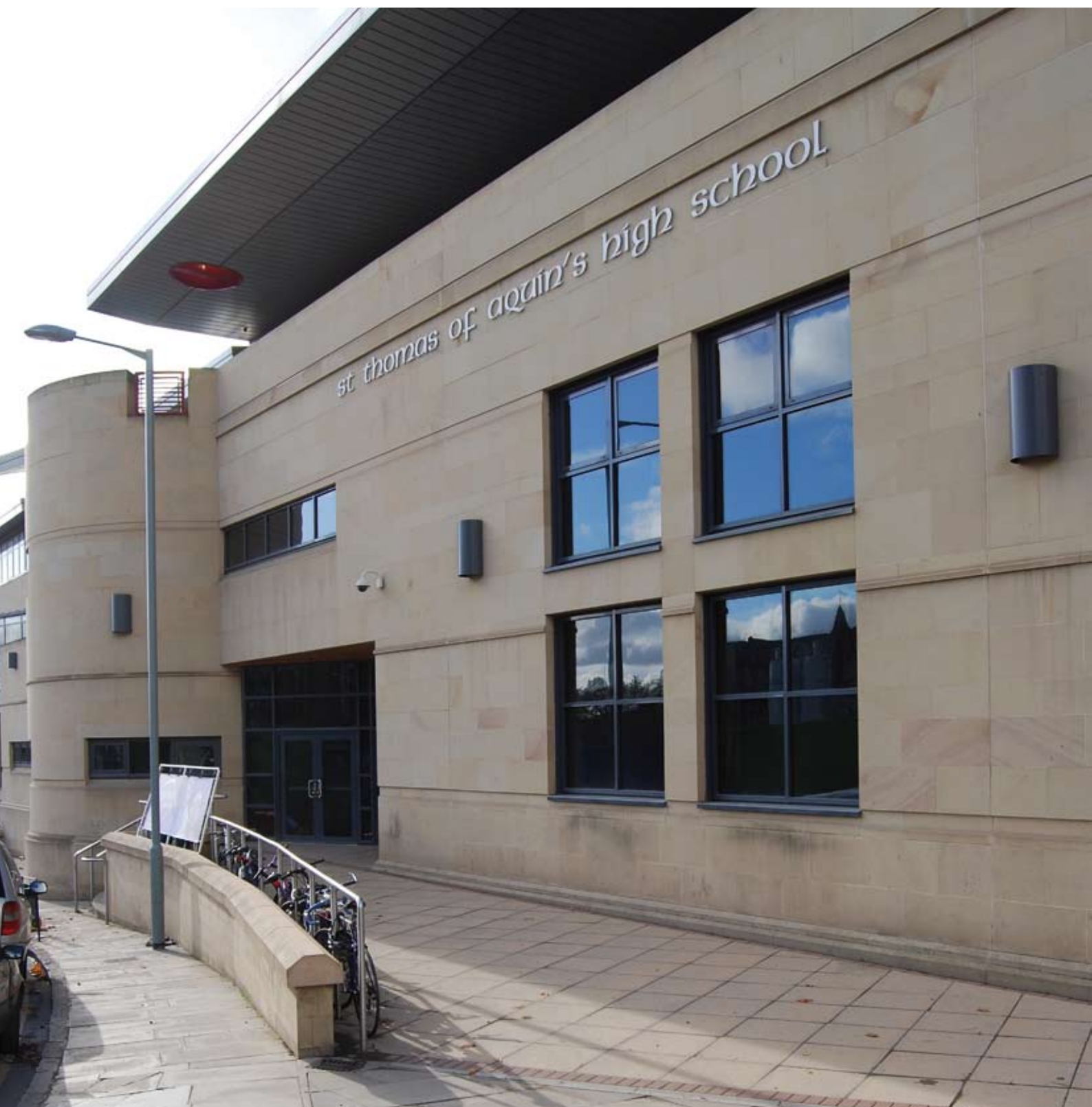
St Thomas of Aquin's High School, Edinburgh. Architect: City of Edinburgh Council.
