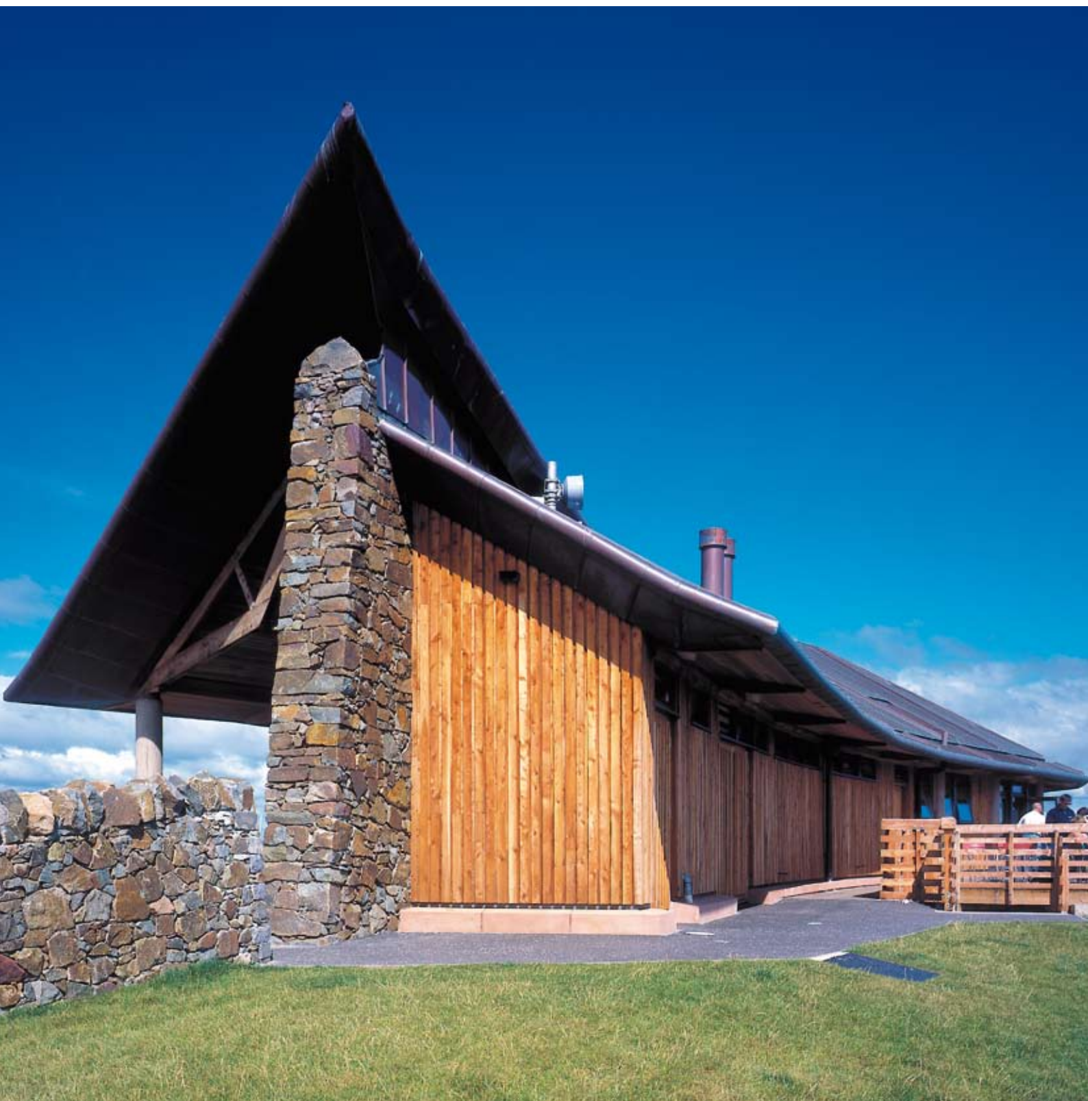
Scottish Seabird Centre, North Berwick. Architect: Simpson & Brown Architects.
