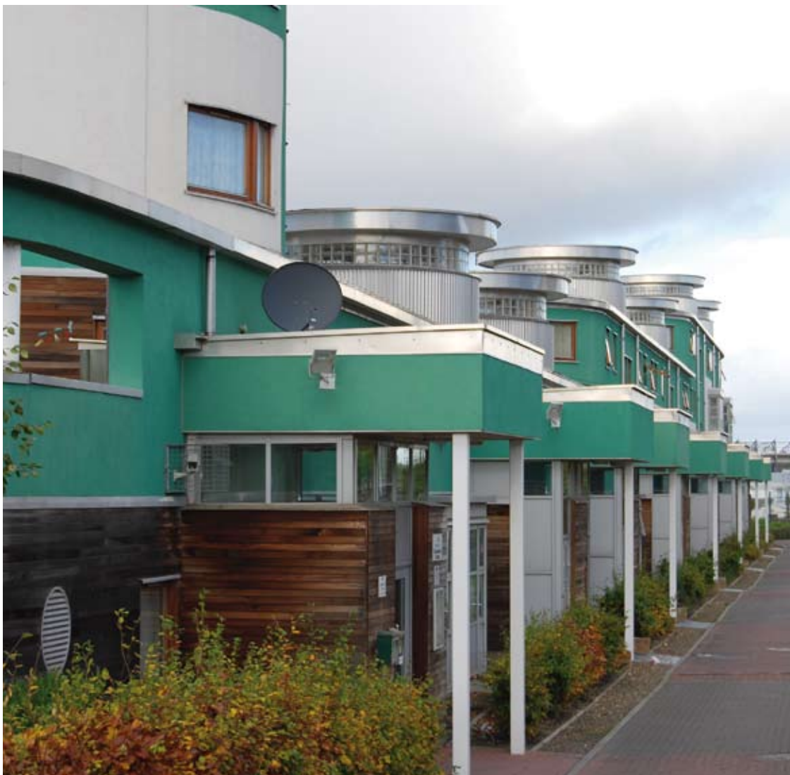
Slateford Housing, Edinburgh. Architect: Hackland & Dore Architects
